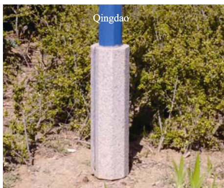
图 8 青岛汇泉广场某碳钢结构的混凝土包覆防腐 Fig.8 Anticorrosion of a carbon steel structure by concrete cover in Huiquan Square, Qingdao
