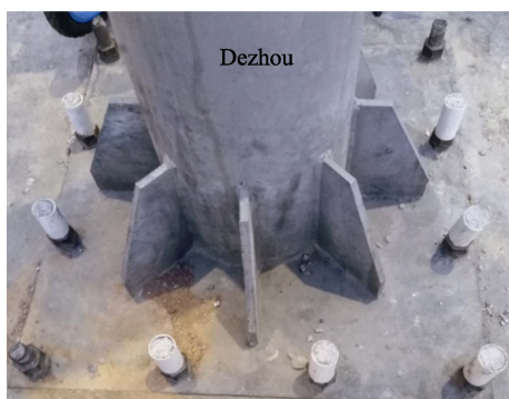
图 12 采用塑料套管灌入混凝土的方法防腐 Fig.12 Corrosion prevention by plastic tubes filled with concrete
