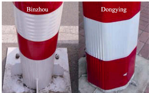
图 6 滨州和东营街道上碳钢结构的玻璃钢包覆防腐 Fig.6 FRP coated anticorrosion of carbon steel structure in streets of Binzhou and Dongying
