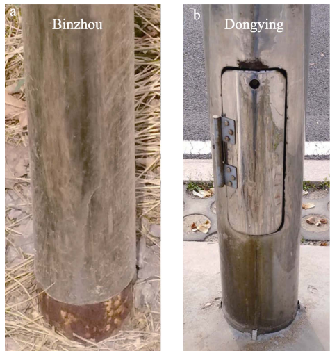
图 7 滨州和东营街道上碳钢结构的不锈钢包覆防腐 Fig.7 Stainless steel covered anticorrosion of carbon steel structure in streets of Binzhou and Dongying
