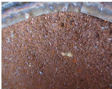
图 3 堵塞的篮式过滤器滤芯 Fig.3 Blocked basket filter element
