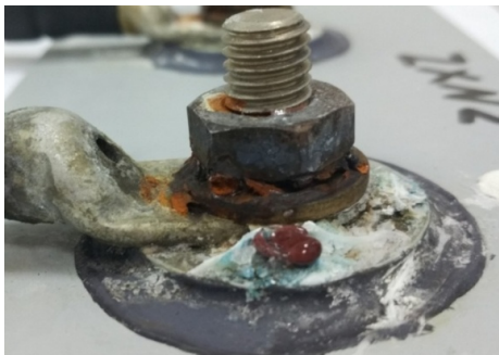
图 7 填角件试验结束后安装板-接地柱间隙形貌 Fig.7 Morphology of gap between mounting plate and ground column after the corner filler test
