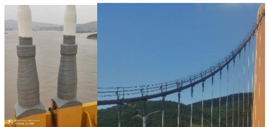
图 7 舟山官山大桥吊杆防水套包覆防腐方案效果 Fig.7 Effect drawing of coating anticorrosion scheme for Suspendor waterproof sleeve of Zhoushan Guanshan Bridge
