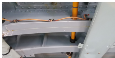
图 1 机身内部承力结构防护涂层的典型外观照片 Fig.1 Typical appearance of the protective coating of the internal load-bearing structure of the fuselage
