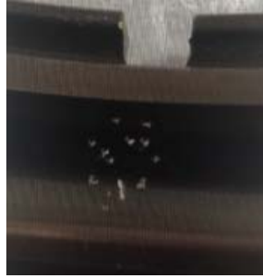
图4 轴承故障细节 Fig.4 Bearing fault details
