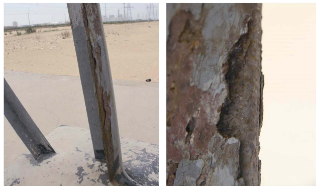
图6 220 kV LL 线塔腿 Fig.6 Tower legs for 220 kV LL transmission line
