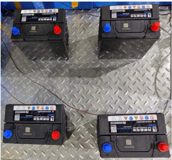
图 2 铅酸蓄电池整体布置及试前检查 Fig.2 Overall arrangement and pre-test inspection of lead-acid battery
